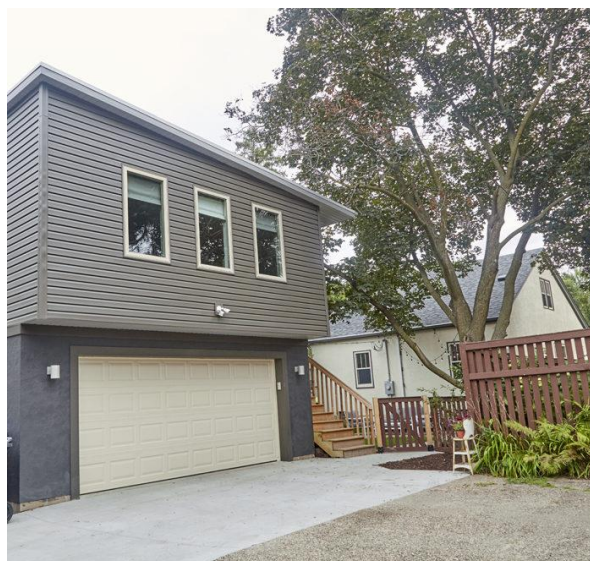
An above-garage ADU in Minneapolis.
